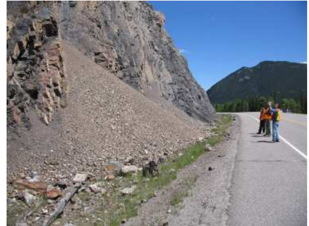
Photo S20-3 – June 2007 (upper left) Facing eastbound along the north highway ditch at the toe of the cut slope. The boulder visible to the right of the Telus pedestal has a maximum dimension of approximately 2 m and was judged to have fallen during 2005 based on the site inspections at that time.
