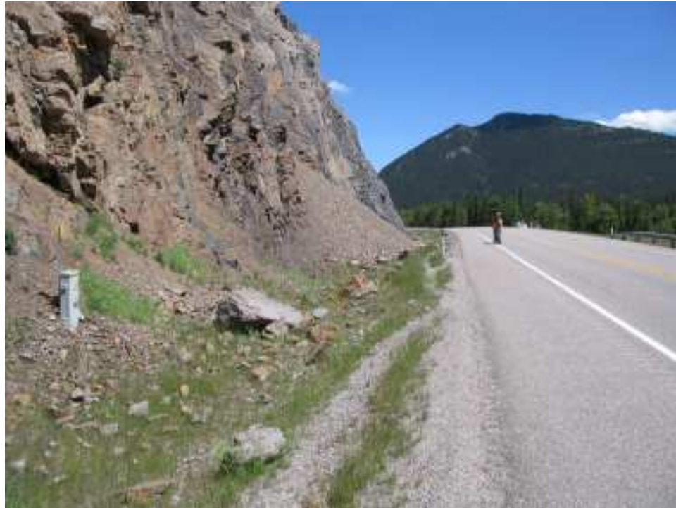
Photo S20-3 – June 2007 (upper left) Facing eastbound along the north highway ditch at the toe of the cut slope. The boulder visible to the right of the Telus pedestal has a maximum dimension of approximately 2 m and was judged to have fallen during 2005 based on the site inspections at that time.
