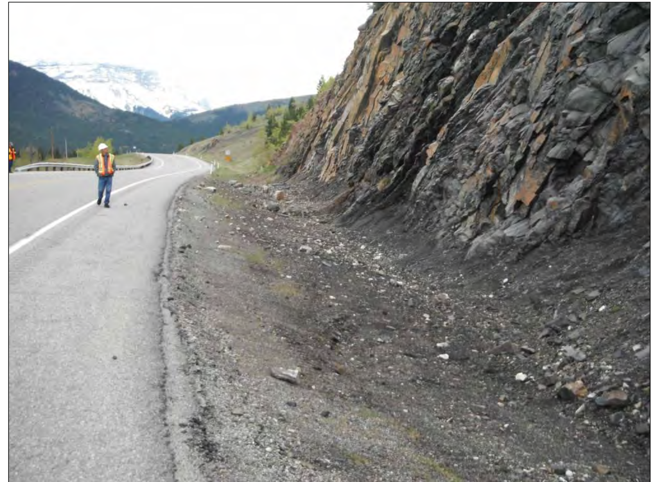
Photograph S20-3 – May 2013
