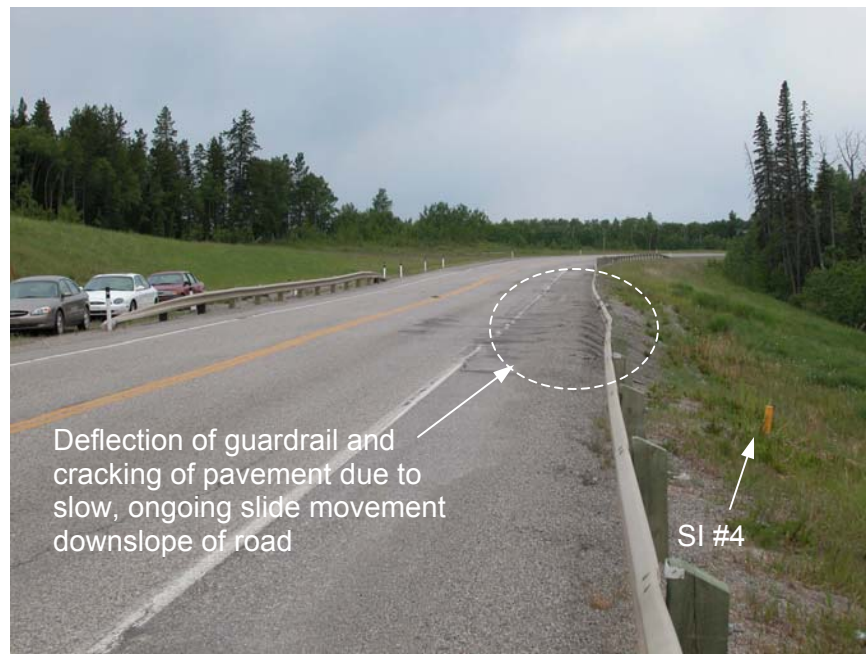
Photo 1 (upper left) – July 2003 Facing west along the downslope edge of the road through the slide area. The existing pile wall is located just to the left of the guardrail. Note the deflection of the guardrail and cracking of the road due to ongoing, slow movement of the landslide below the road – appears to be worse than noted in May 2002 (Photo 2). The north shoulder of the road (adjacent to the guardrail) required patching in the summer of 2002 and was scheduled for repaving again later in the day that this photo was taken (July 8, 2003).
