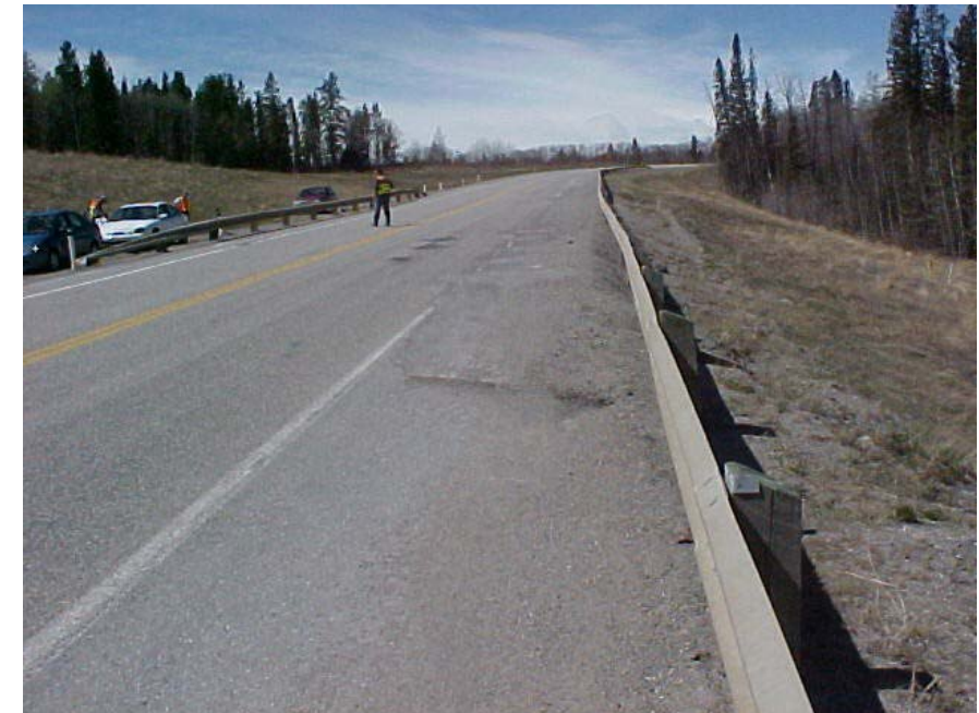
Photo 1 (upper left) – July 2003 Facing west along the downslope edge of the road through the slide area. The existing pile wall is located just to the left of the guardrail. Note the deflection of the guardrail and cracking of the road due to ongoing, slow movement of the landslide below the road – appears to be worse than noted in May 2002 (Photo 2). The north shoulder of the road (adjacent to the guardrail) required patching in the summer of 2002 and was scheduled for repaving again later in the day that this photo was taken (July 8, 2003).
