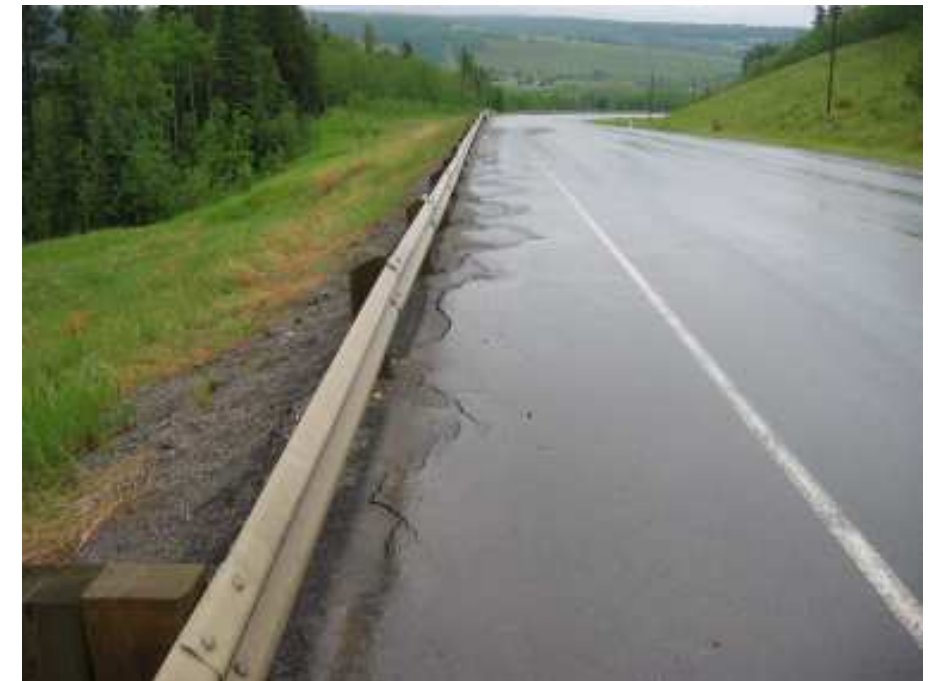
Photo S2-1 (upper left) – June 2005 – Cracking in the westbound lane. Cracking developed between the time of the instrument readings in May 2005 and the annual inspection in June 2005. Based on the pattern of the cracks and settlement down to the north (right hand side of photo), it appears that the existing pile wall is resisting slope movement downslope of the road.
