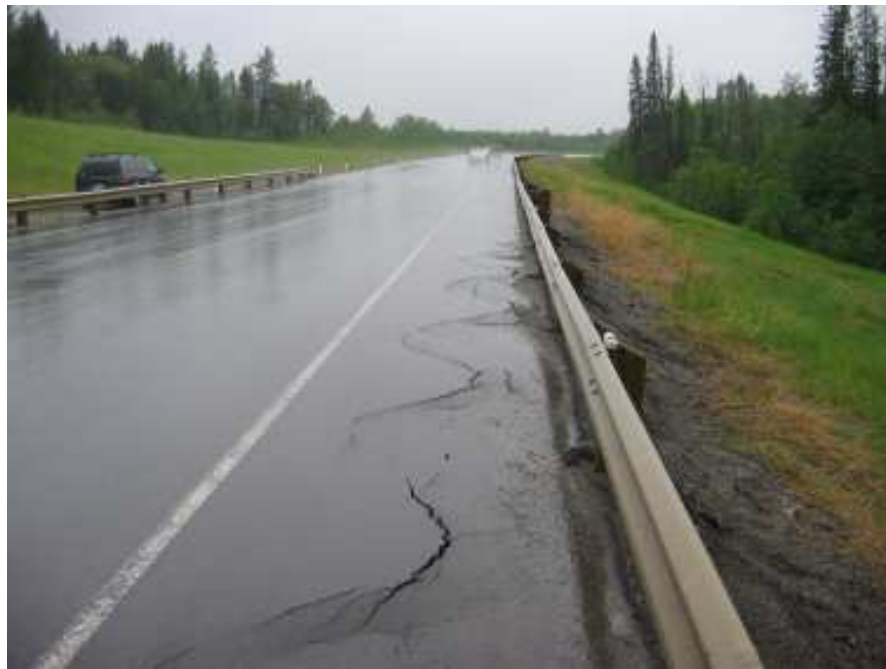
Photo S2-1 (upper left) – June 2005 – Cracking in the westbound lane. Cracking developed between the time of the instrument readings in May 2005 and the annual inspection in June 2005. Based on the pattern of the cracks and settlement down to the north (right hand side of photo), it appears that the existing pile wall is resisting slope movement downslope of the road.
