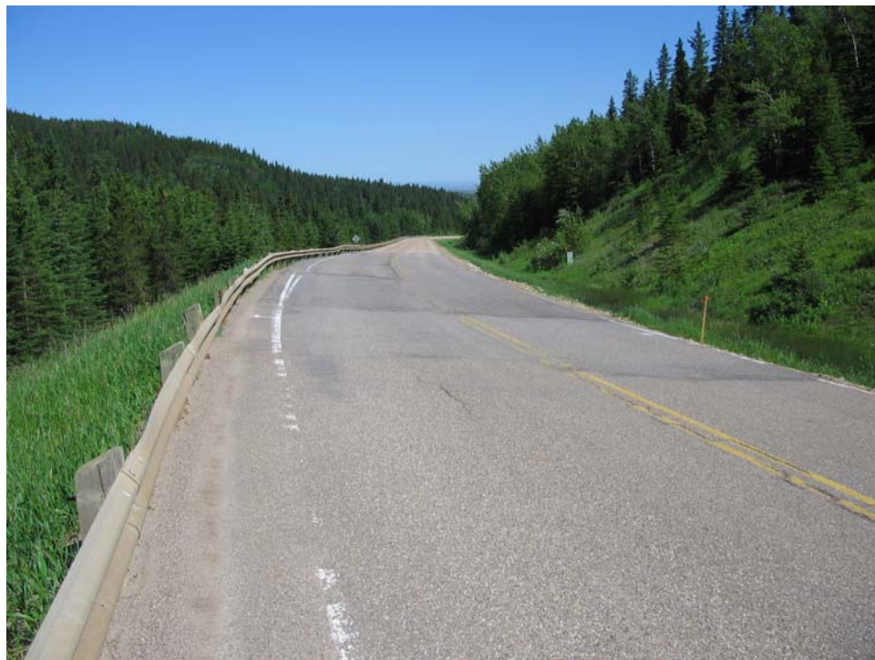
Photo S26-4 – June 2007 (bottom left) Facing northbound along the segment of highway shown in Photo S26-3. Note the bumps and dips in the road grade due to landslide damage.
