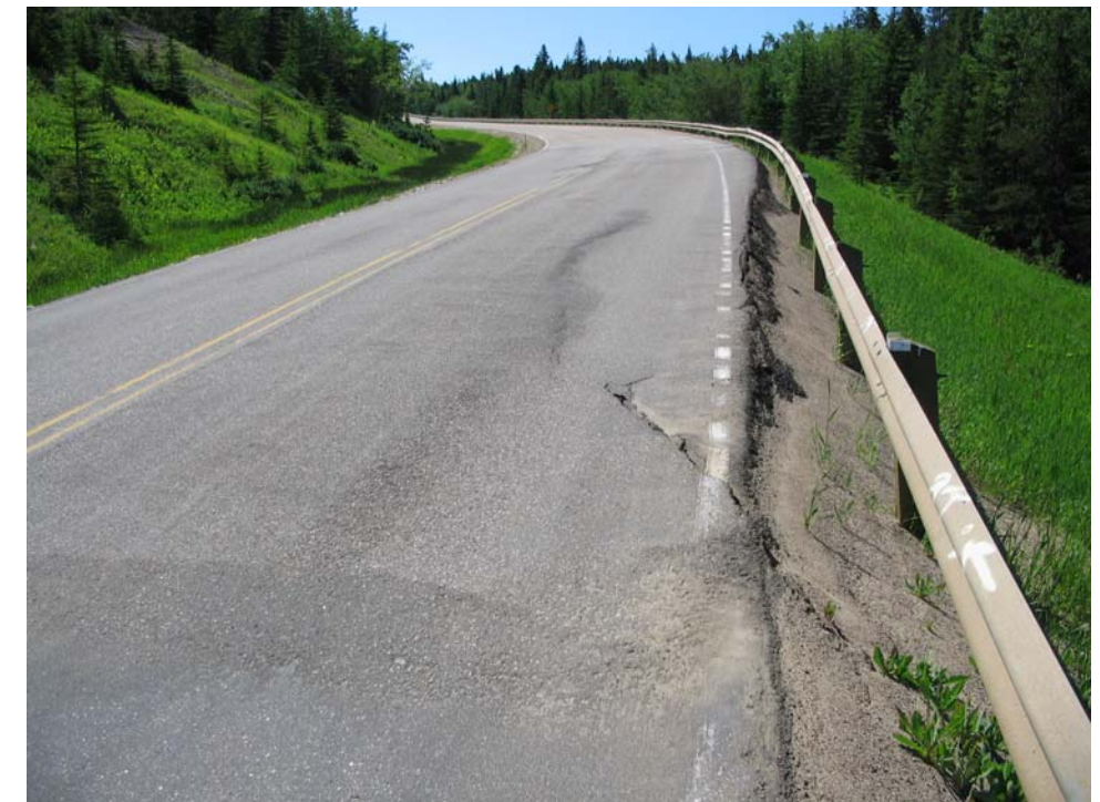
Photo S26-4 – June 2007 (bottom left) Facing northbound along the segment of highway shown in Photo S26-3. Note the bumps and dips in the road grade due to landslide damage.
