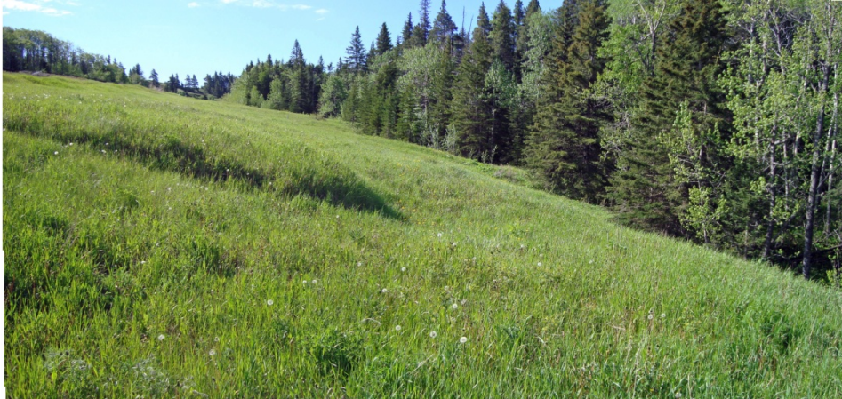
Photo S26-6 – top - (June 2011) A slump on the lower slope at Area A, in much the same condition as was observed during the June 2010 inspection.
