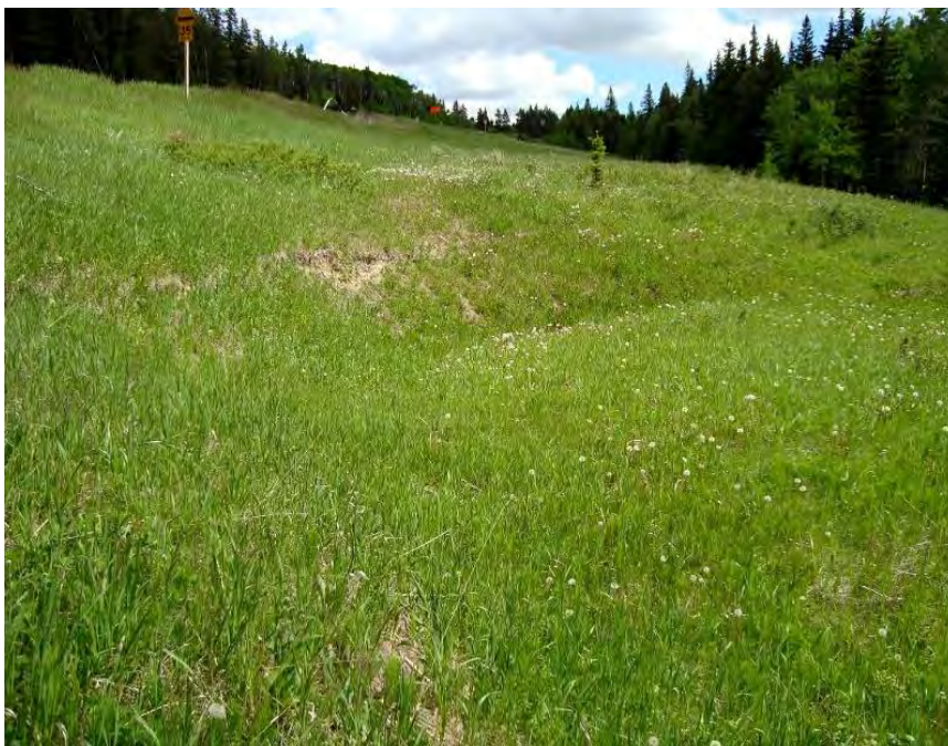
Photo S26-2 - (June 2012) Facing south from the north end of Area A at the lower west slope. Fresh soil was exposed at the headscarp of one of the main lower slides.
