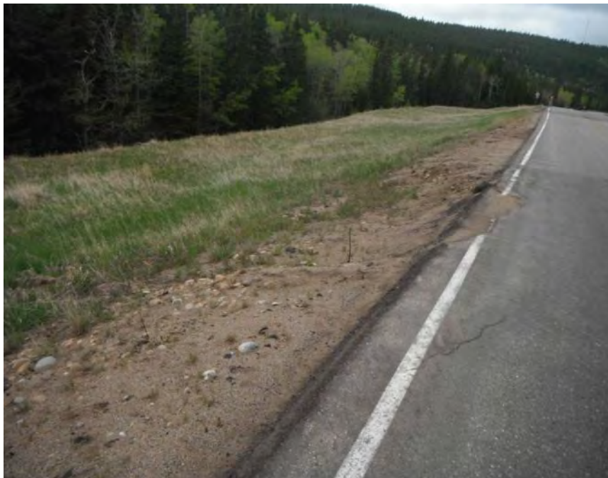
Photo S26-2 - (May 2013) Facing northwest from the south end of Area A at the west road shoulder. Overlays have been placed at the damaged areas in Fall 2012. Minor cracking and settlement was visible along the shoulder through the new overlay.
