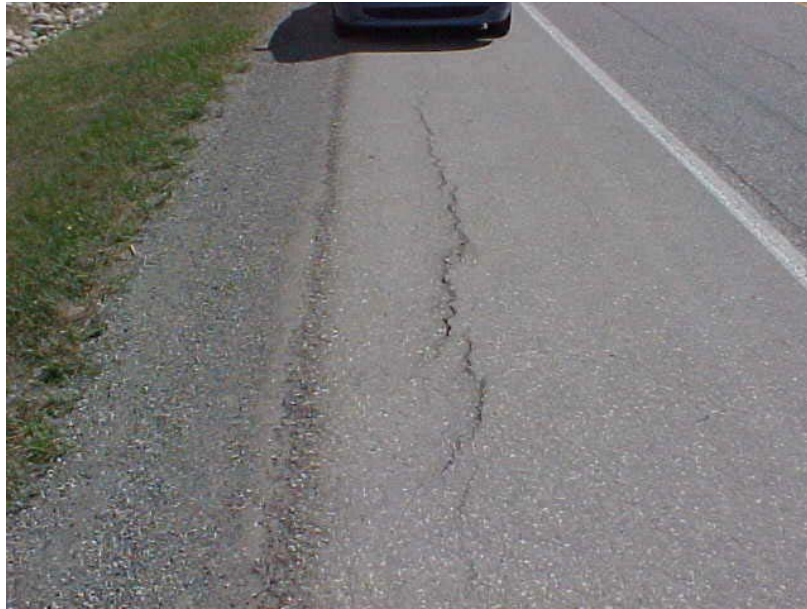
Photo 3 – Close up view of cracking on north shoulder of road adjacent to SI #4.
