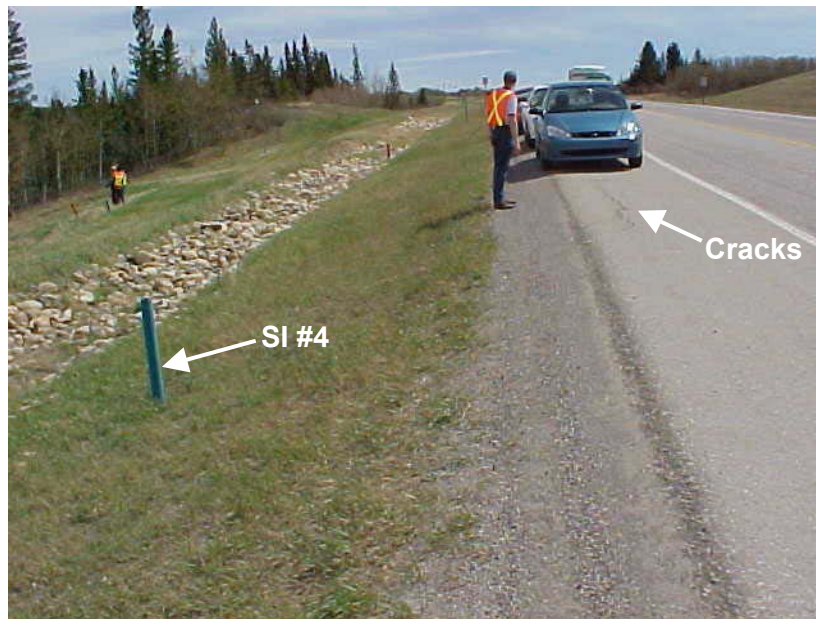
Photo 2 – Cracking on north shoulder of road adjacent to SI #4 (blue casing on left of photo). The cracking appeared to be longitudinal, but could possibly be associated with continued downslope movement at approximately 2.7 m depth in SI #4.
