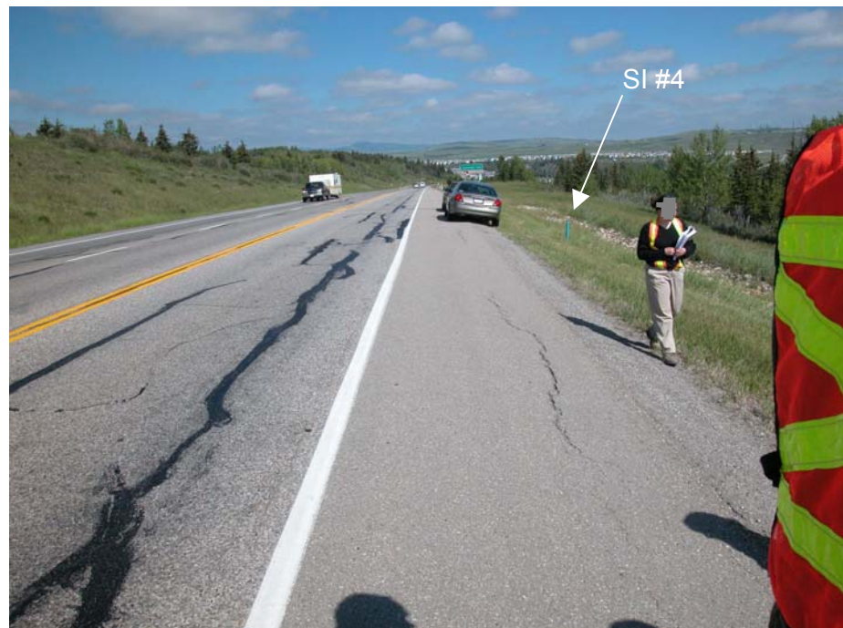
Photo 4 (lower right) – July 2003 Another view of the crack adjacent to SI #2 that has developed since the May 2002 inspection.
