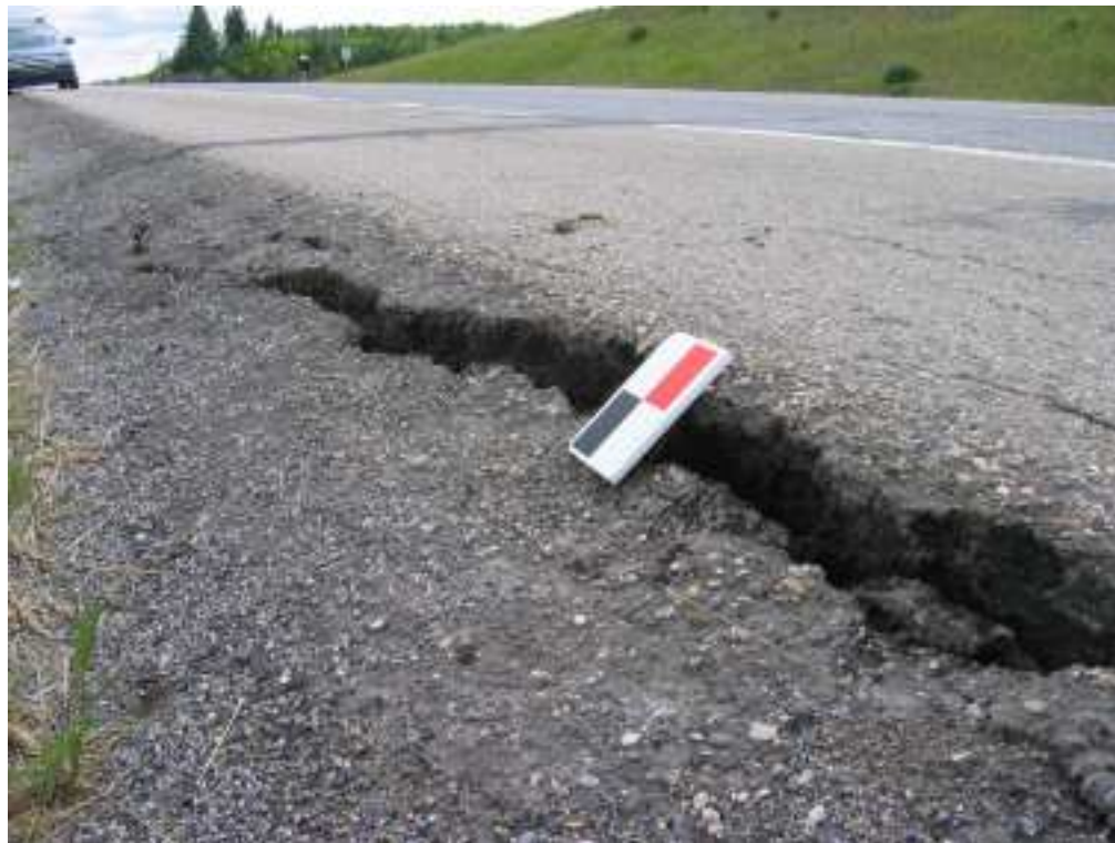
Photo S3-5 (lower left) – June 2005 – closer view of recent cracking in westbound shoulder. Field notebook for scale.
