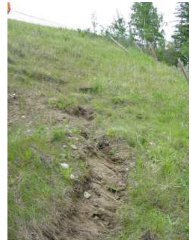
Photo S3-3 (lower right) – June 2005 – shallow sloughing on slope to the north of the road. This particular feature was new this year and most likely developed during heavy rainfall in mid to late June 2005.
