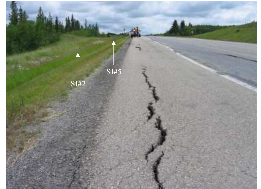
Photo S3-5 (lower left) – June 2005 – closer view of recent cracking in westbound shoulder. Field notebook for scale.
