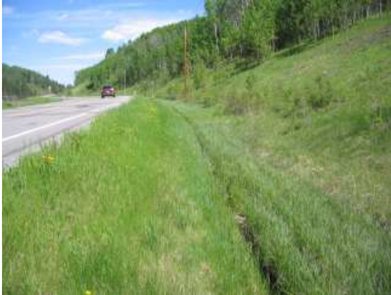
Photo S31-5 (top) – June 2008 Facing north along the upslope ditch. There was clear water flowing southwards in the wheel ruts in the ditch. There did not appear to be a specific source location for the water. The inlet of the culvert at the site could not be found in the ditch.
