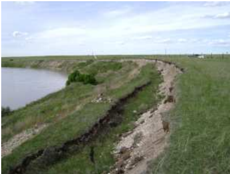
Photo S32-2 (bottom) – June 2008 Facing north/upriver across the landsliding area along the outside of the meander bed in the river channel. The cars visible in the right background of this photo are parked on far side of the highway (Photo S32-1).
