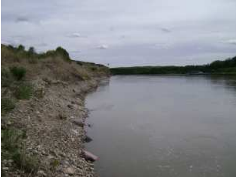
Photo S32-5 (top) – June 2008 Facing downriver along the left (east) bank erosion area along the outside of the meander bend in the channel.
