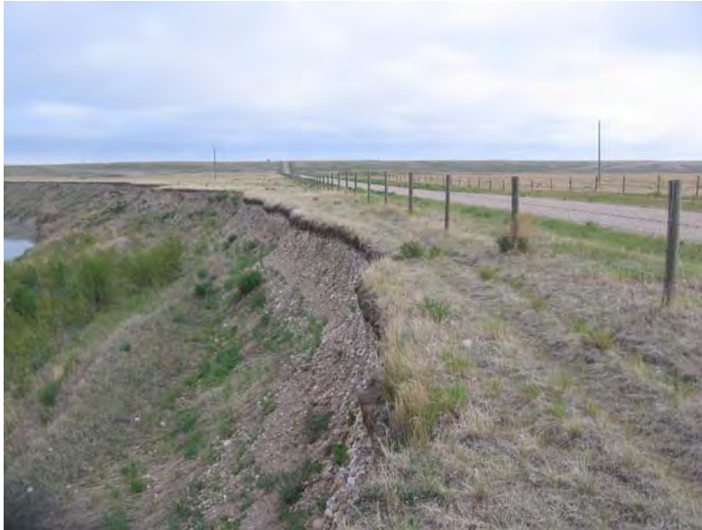
Photo S32-1 (top) – June 2009 Facing north along the highway, adjacent to the bank erosion and slope instability. The Bow River channel is visible on the left side of the photo.
