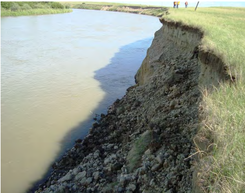
Photo S32-2 – June 2012 Facing south towards the area near the ferry sign where fresh bank retrogression was observed.
