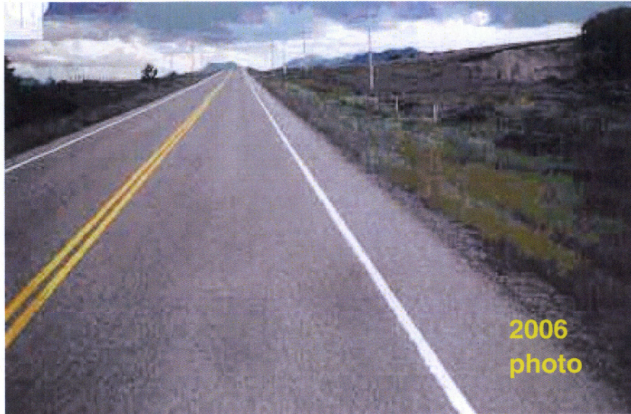
Photo 7 (top) – Photo from 2006 videolog provided by AT, facing southbound along the highway adjacent to the landslide area. Note the significantly greater offset between the crest of the slope and the highway compared to the June 2009 photos.
