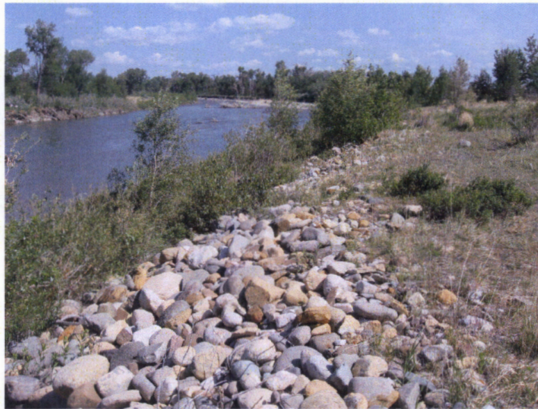
Photo 5 (top) – View downstream of the armored right bank, which is located downstream of the meander bend and landslide area. The upstream end of this armored segment of the bank is being outflanked and eroded by the meander bend.
