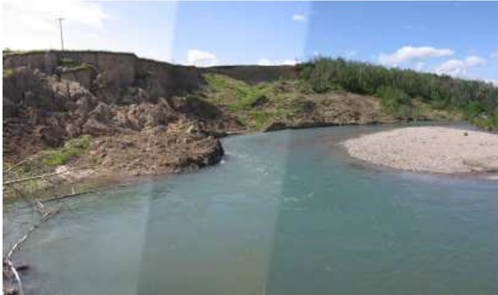
Photo 3 (top) – View upstream towards the toe of the landslide area. Photo is taken from the downstream end of the meander loop and on top of the armored right bank downstream of the landslide area that is being outflanked and eroded. Note the significant toe bulge/thrust from the recent landsliding.
