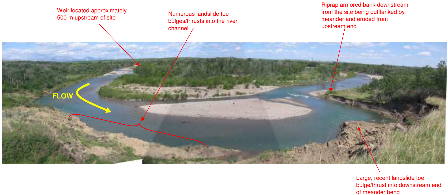
Photo 1 – View from the crest of the slope above the landslide area, a short distance south/upstream from the area of significant retrogression towards the highway in recent years. The sharp bend in the river channel immediately upstream of the site is evident, along with the meander in the channel that directly attacks the toe of the slope in the landslide area. Figure 1 contains further annotations illustrating the site features shown above.
