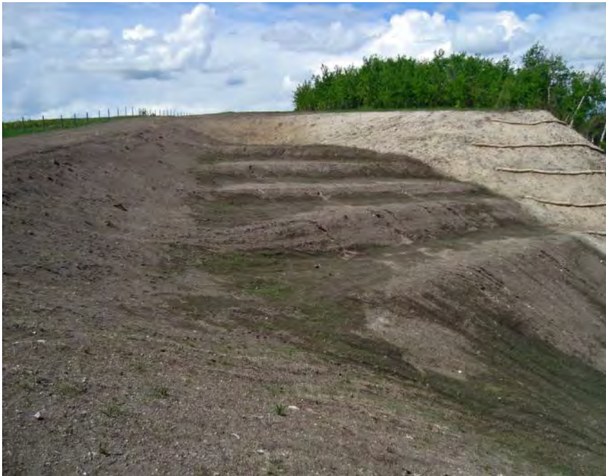
Photo S36-3 - (May 2013) Standing near the top of the graded slope looking towards the south at the borrow area. Minor vegetation growth and rilling on the benches was visible.
