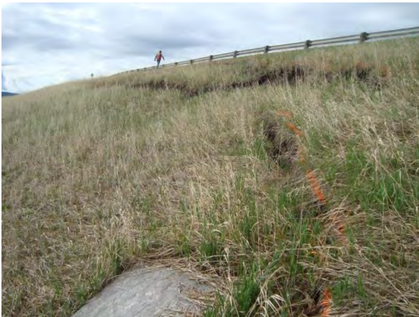
Photo S38-2 (May 2013) Sliding near the north end of the site. The main scarp is marked in orange on the photo.
