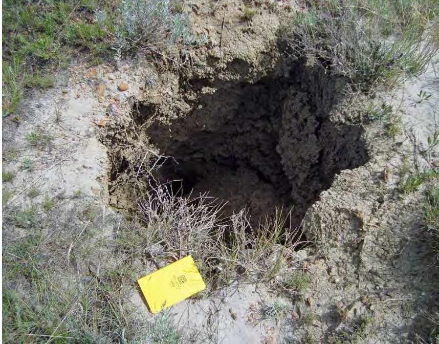
Photo S40-2 – June 22, 2012 One of several typical sinkhole features found throughout the site area. This particular sinkhole was located at reference point 97 on Figure S40-1.
