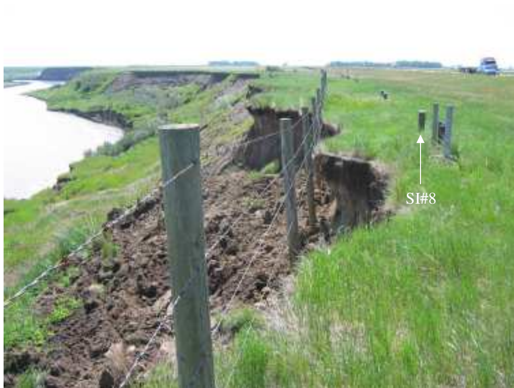
Photo S4-3 (lower left) – June 2005 – facing south across the area where the landslide scarp has retrogressed across the fenceline since the 2004 inspection.
