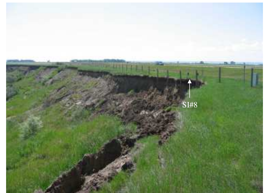
Photo S4-3 (lower left) – June 2005 – facing south across the area where the landslide scarp has retrogressed across the fenceline since the 2004 inspection.
