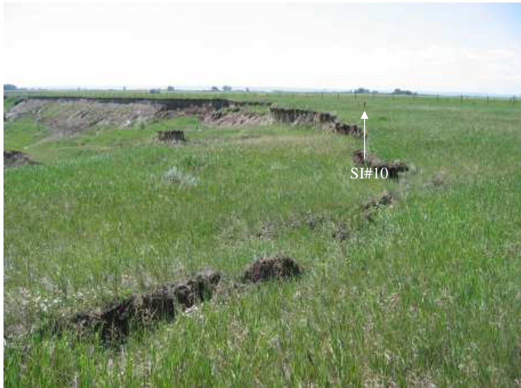
Photo S4-5 (upper left) – June 2005 – recent downdrop of landslide block along the northern flank of the landslide area.
