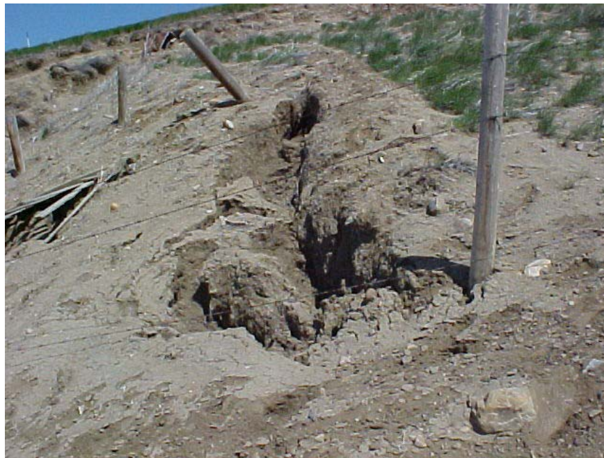
Photo 3 – Recent gullying and piping in the exposed soils on the landslide blocks immediately downslope of the road.
