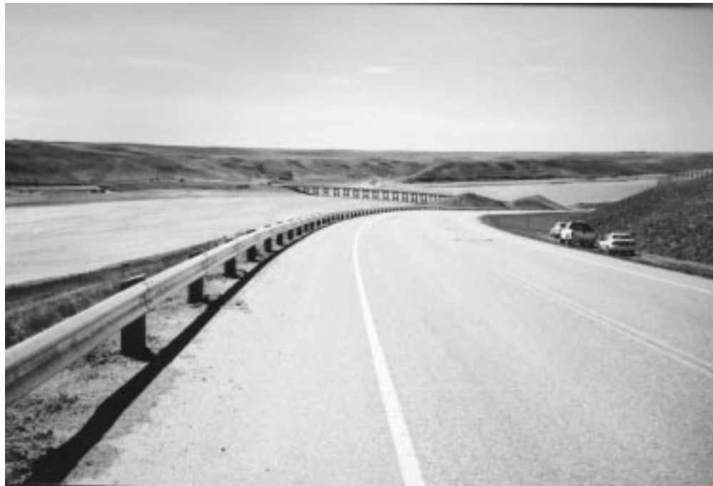
Photo 4 – Facing southwest along road through slide area. Note newly-installed guardrail.
