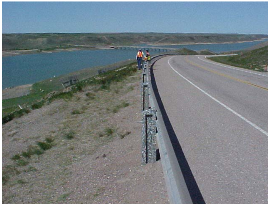
Photo 4 (lower right) July 2003 Facing east across the recent shallow slumping area. The road surface has not been damaged, despite the proximity of the slumping.
