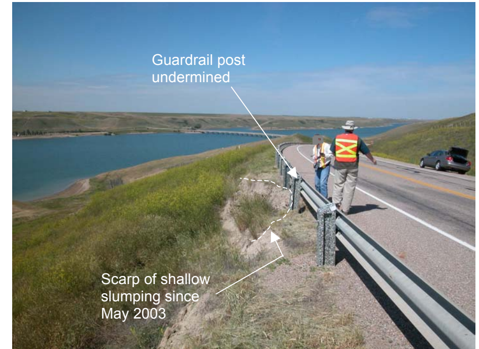
Photo 2 (upper right) July 2003 Closer view of the area where shallow slumping occurred along the scarp of the slide area. One of the guardrail posts has been undermined by the movement, and the two adjacent posts are very close to becoming undermined.
