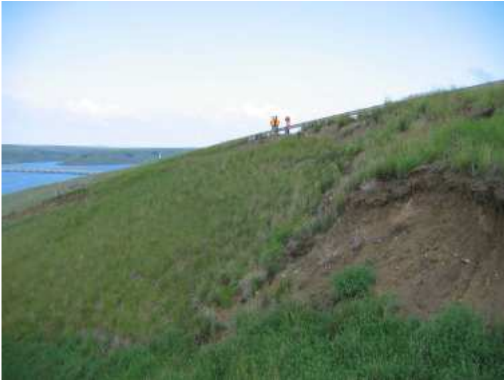
Photo S5-4 (left) – shallow slumping on slope downslope of the road.
