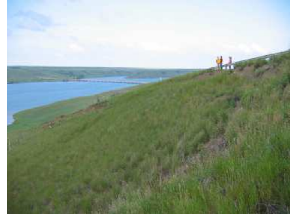
Photo S5-1 (upper left) – June 2005 – facing east across the shallow slumping area that is undermining the guardrail along the downslope edge of the road. Possible additional cracking since the 2004 inspection was noted but the overall state of the slumping did not appear to have changed significantly.
