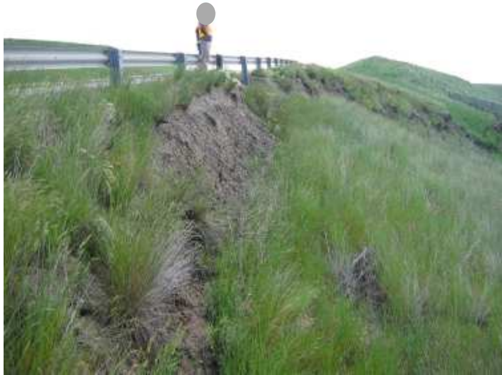
Photo S5-1 (upper left) – June 2005 – facing east across the shallow slumping area that is undermining the guardrail along the downslope edge of the road. Possible additional cracking since the 2004 inspection was noted but the overall state of the slumping did not appear to have changed significantly.
