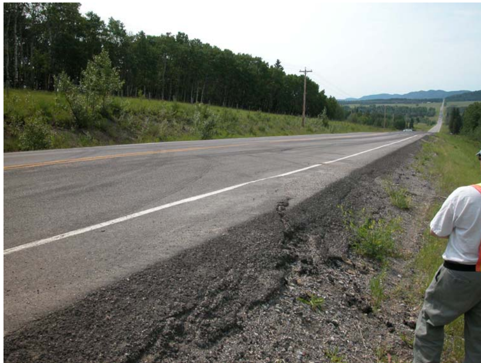
Photo 1 (upper left) Facing south across the settlement and cracking area at the north end of the site. The cracking and settlement in this area has not changed significantly since the May 2002 inspection.
