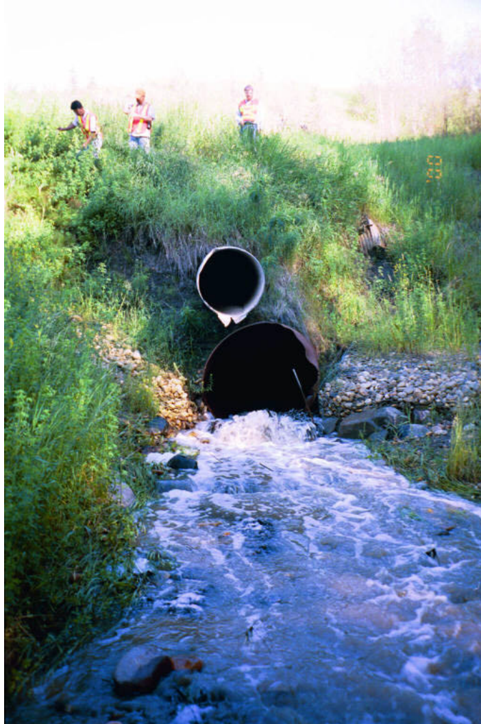
Photo 1: Whitemud River, culvert outlet, 2000
