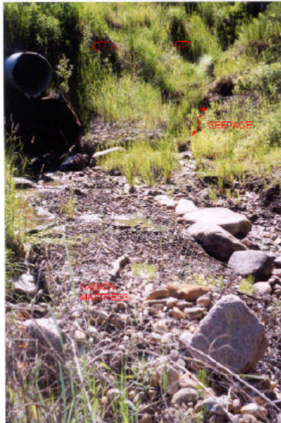
Photo 2: Whitemud River, culvert outlet, 2001
