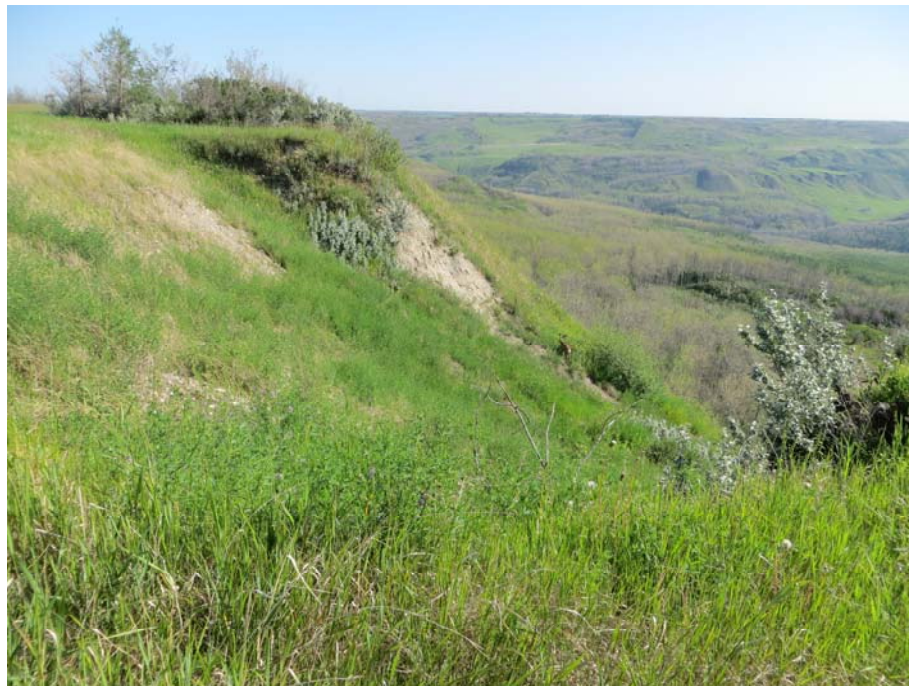
Photo 2. No significant change in the backscarp of Slide 1 since 2011 – the repair continues to be effective.
