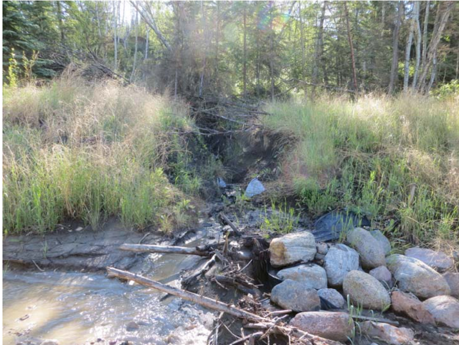
Photo 4 - Looking east at a 10 m long x 1.5 m deep erosion gully that has enlarged on the east side of the channel in front of the culvert inlet.
