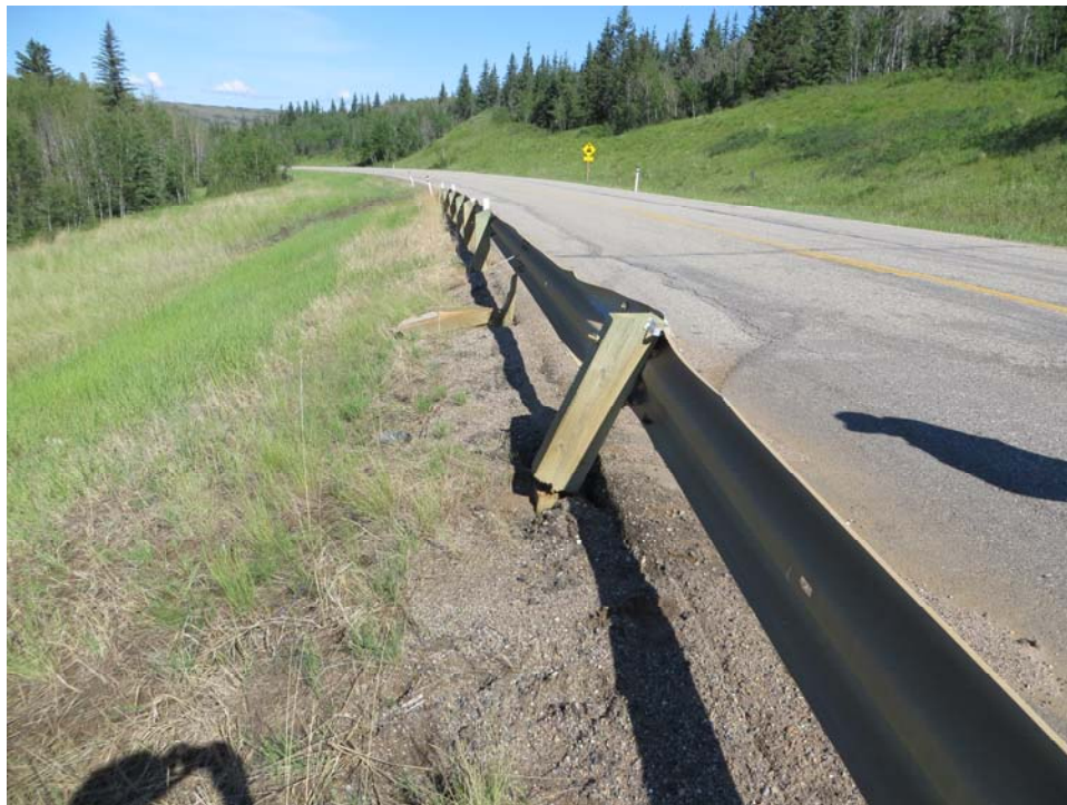
Photo 8 - Looking west along the south guardrail that is damaged.
