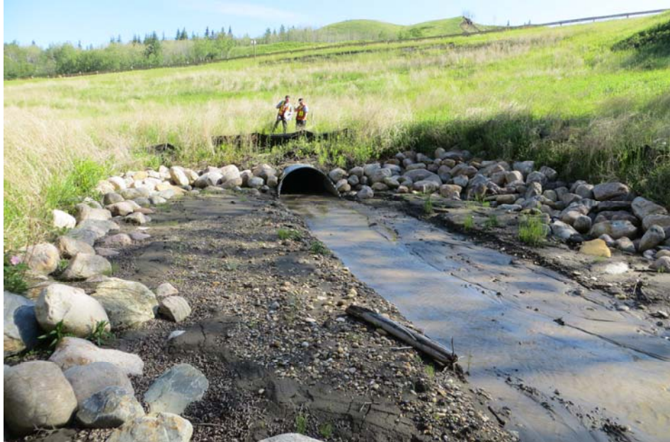
Photo 7 - Looking northwest at the new culvert outlet. It is about 50% full of sediment.
