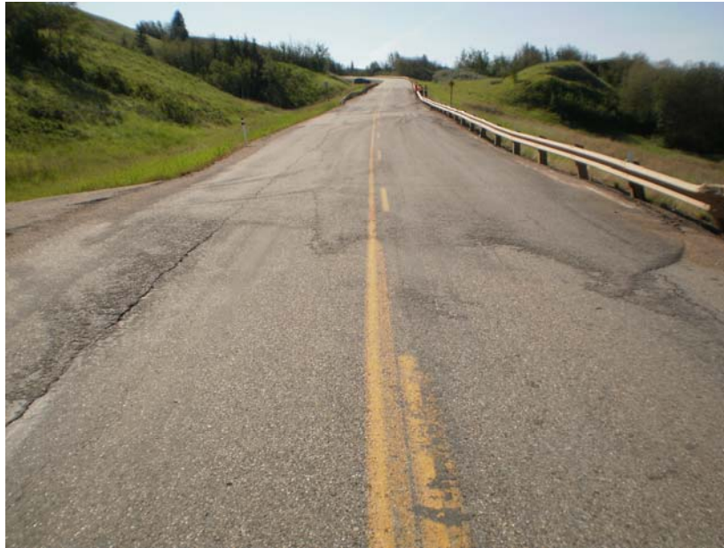
Photo 1 - Looking east along the highway over the Grimms Creek site area. Note the ACP patches and the dip in the highway.
