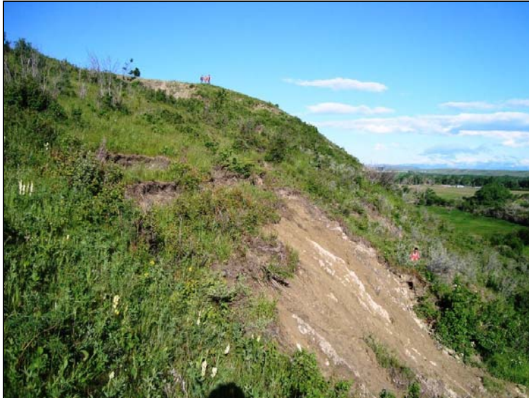
Photo 5 (June 21, 2011) Facing west at an active secondary scarp on the slide mass. A large increment of movement occurred here recently. Slide activity appears to extend to a bedrock outcropping slightly below this location.
