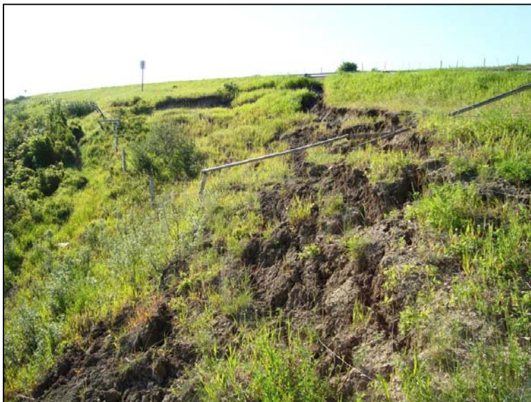
Photo 4 (June 21, 2011) Facing southeast from the west flank of the landslide. Recent slide activity is visible (note also the displaced fenceline)
