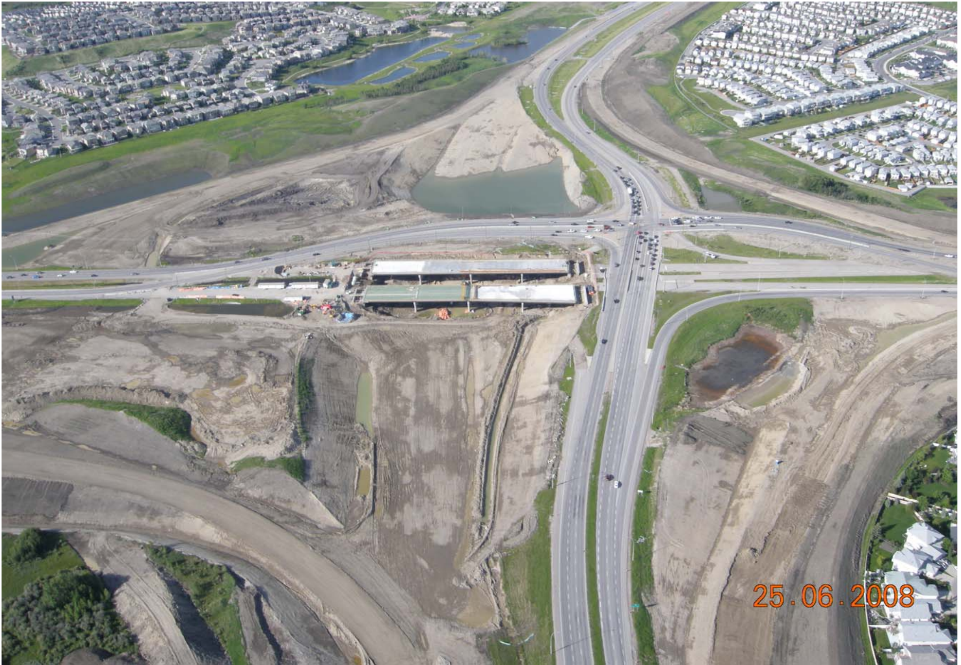
Stoney Trail / Crowchild Trail Interchange Looking North June 2008
