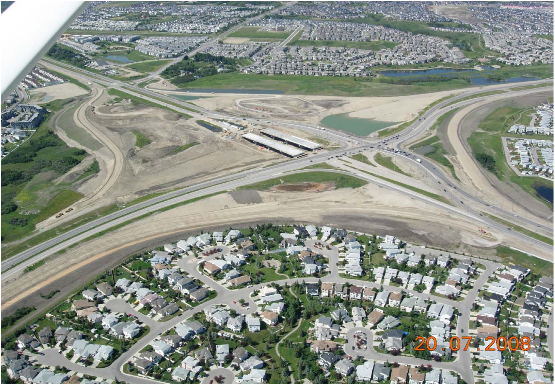
Stoney Trail / Crowchild Trail Interchange Looking North July 2008
