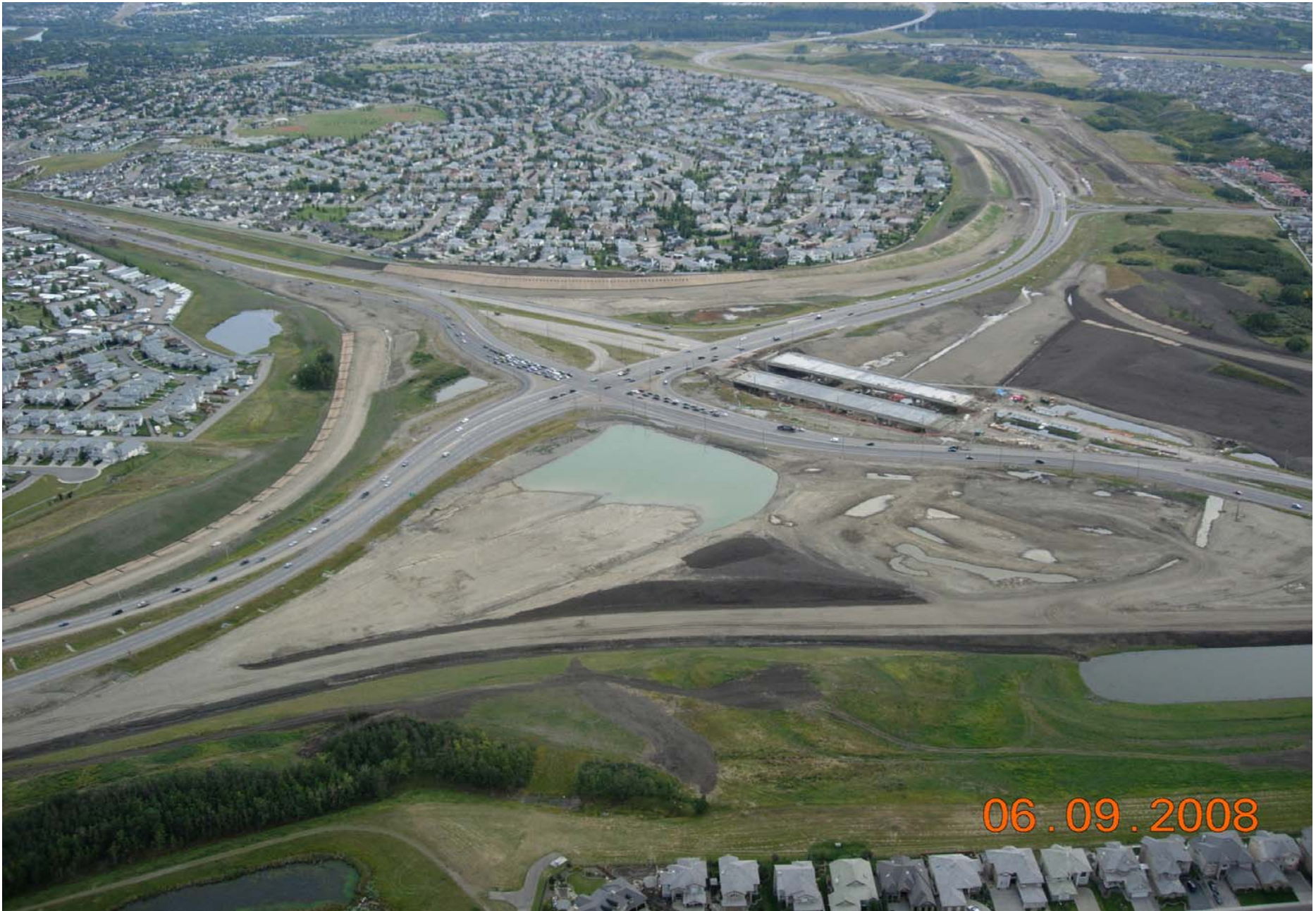
Stoney Trail / Crowchild Trail Interchange Looking Southeast September 2008
