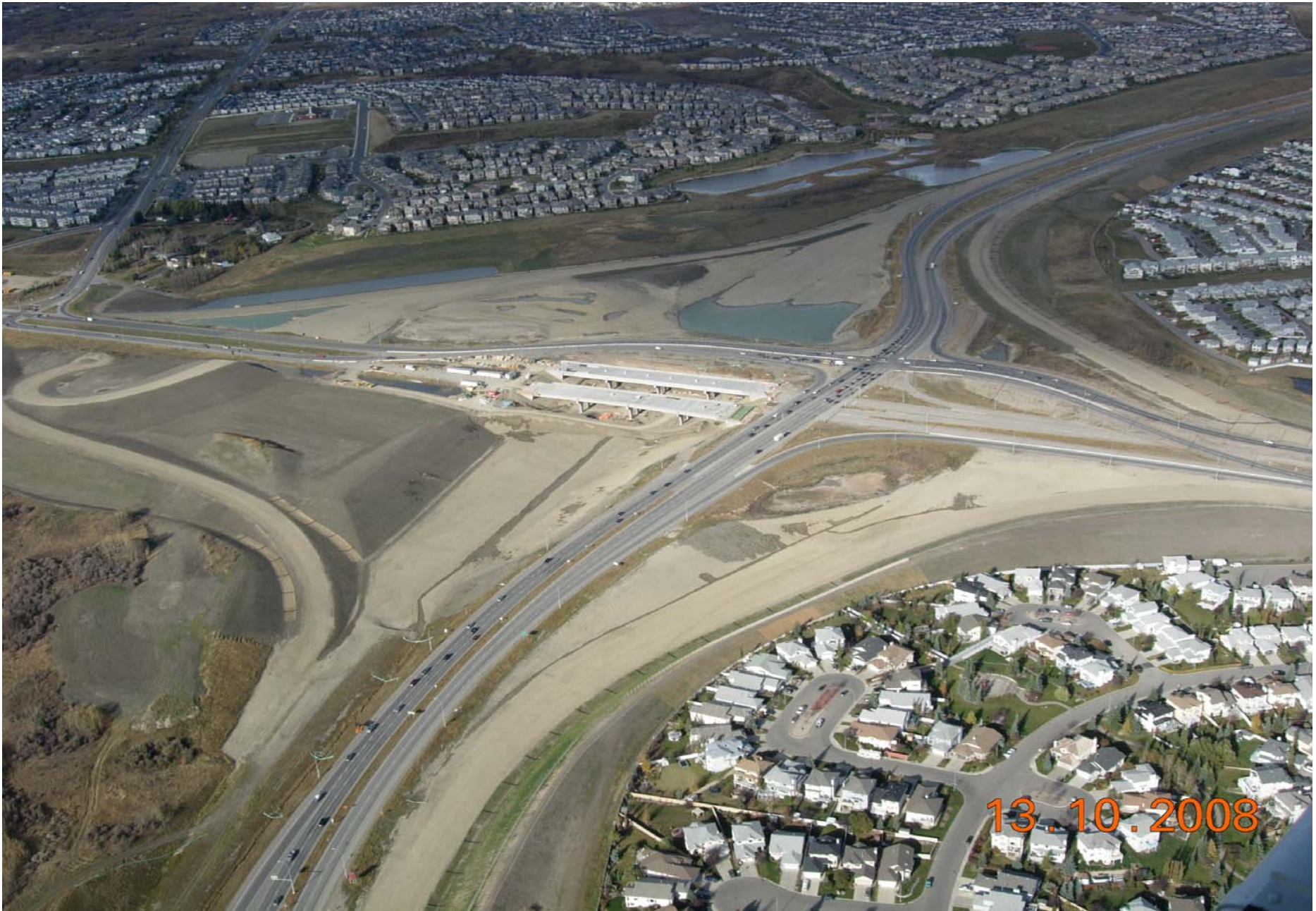
Stoney Trail / Crowchild Trail Interchange Looking North October 2008
