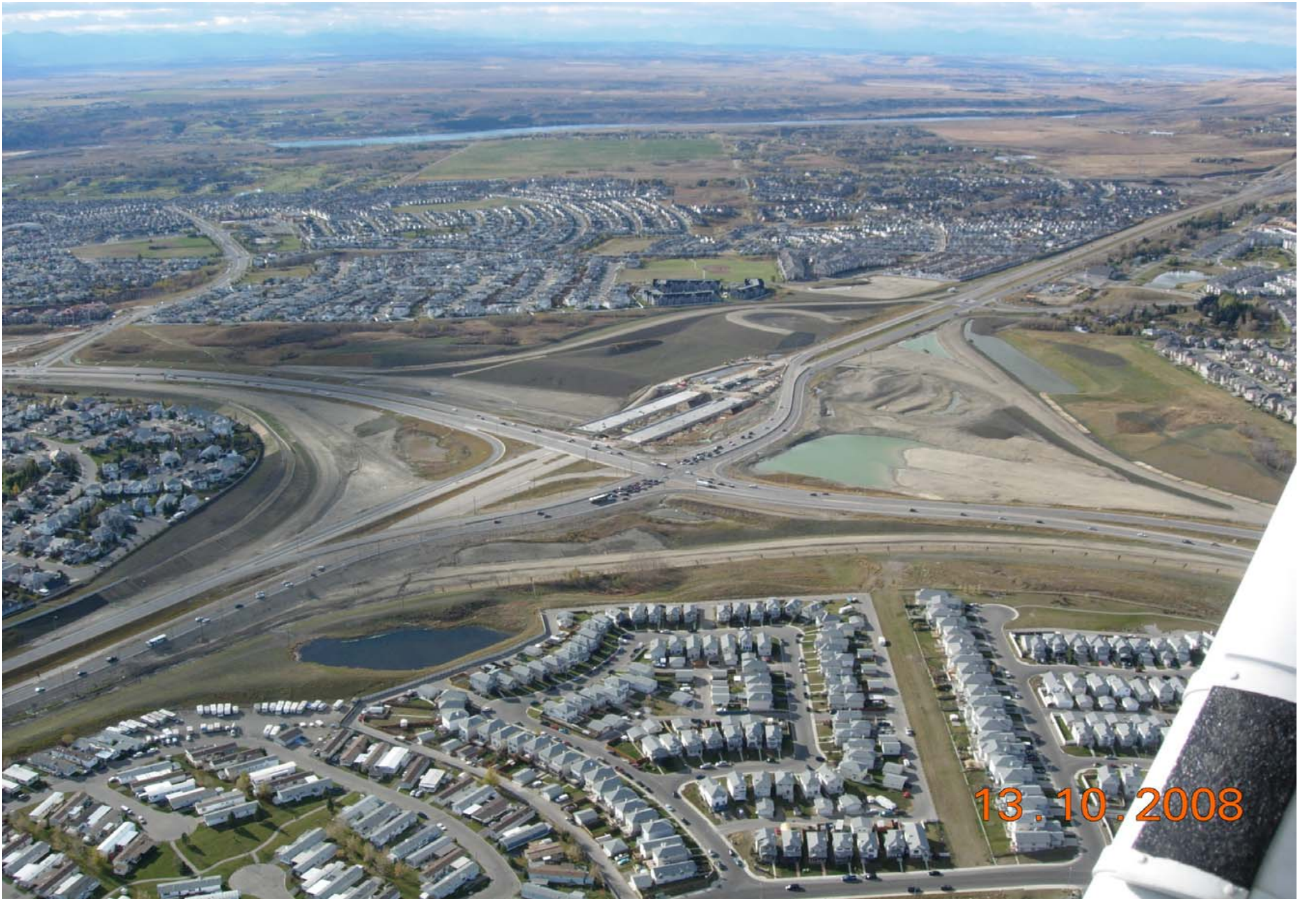
Stoney Trail / Crowchild Trail Interchange Looking Southwest October 2008
