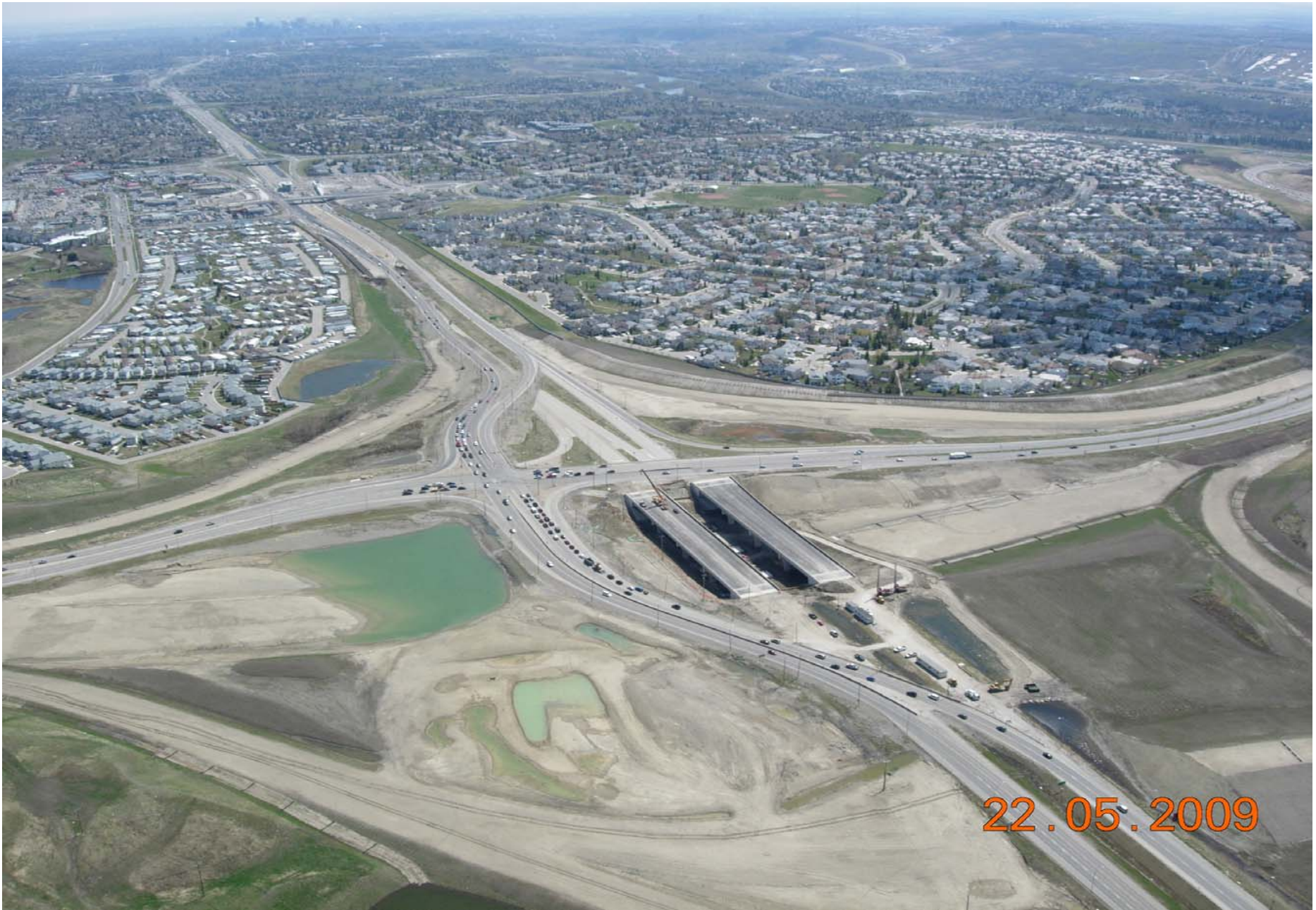
Stoney Trail / Crowchild Trail Interchange Looking Southeast May 2009
