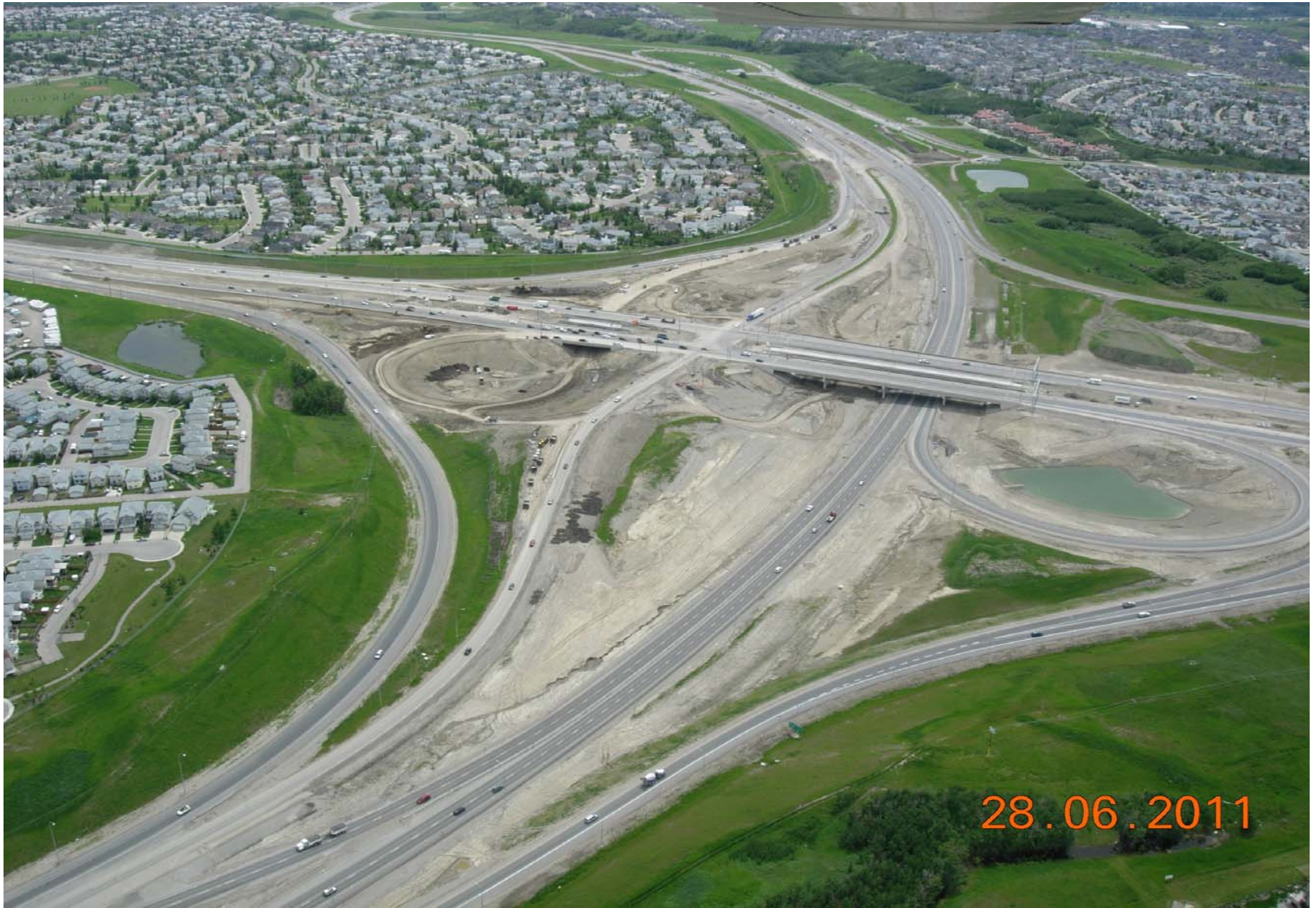
Stoney Trail / Crowchild Trail Interchange Looking Southeast June 2011
