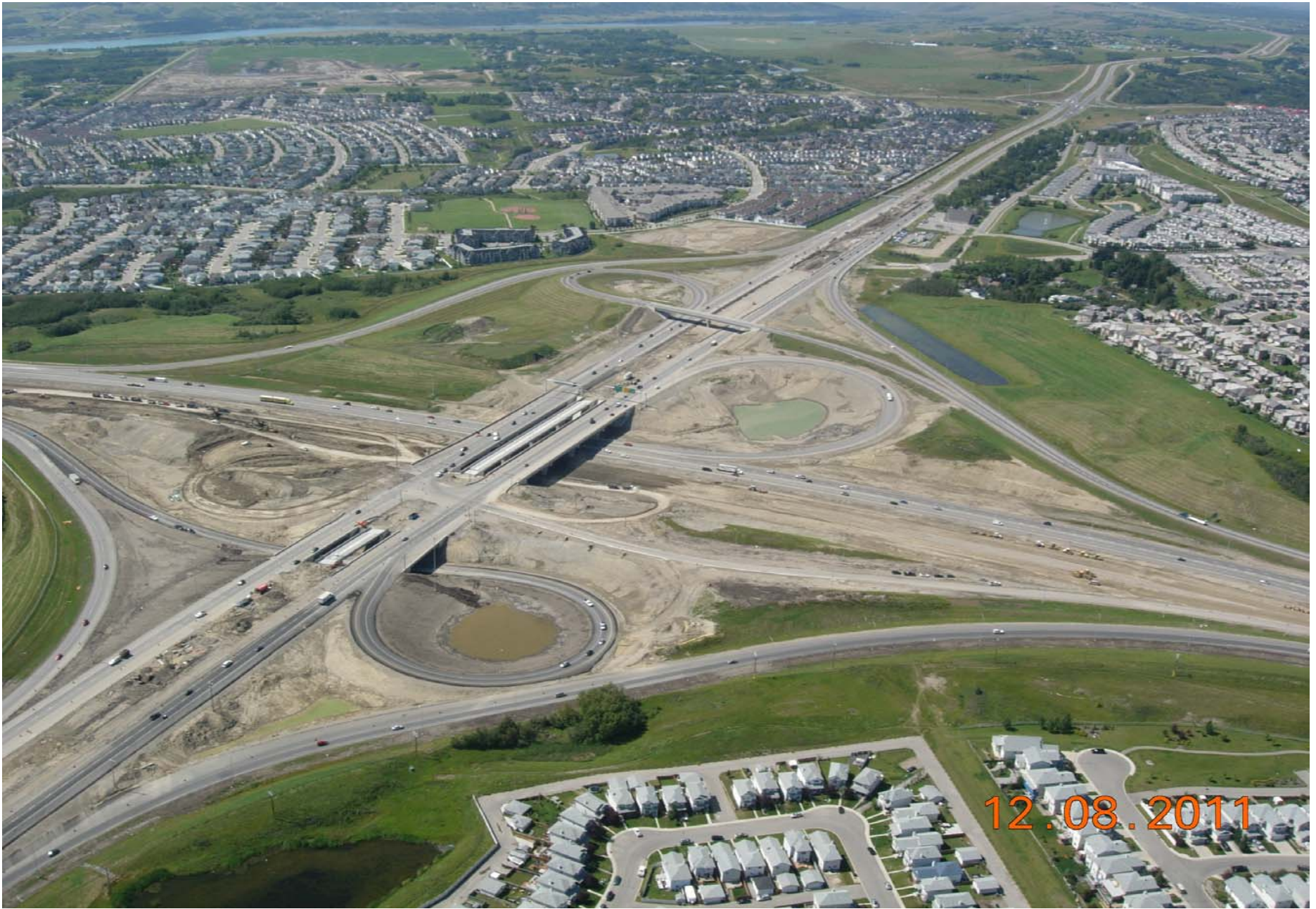
Stoney Trail / Crowchild Trail Interchange Looking Southwest August 2011
