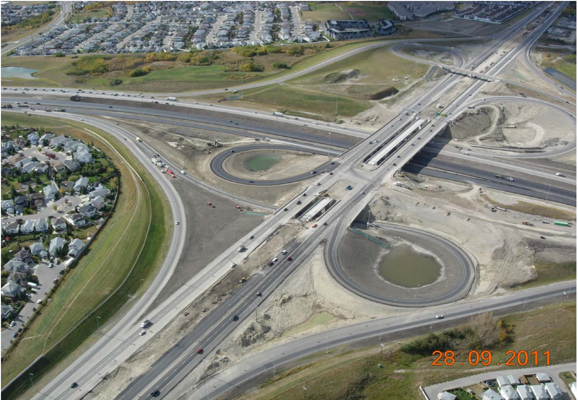
Stoney Trail / Crowchild Trail Interchange Looking Southwest September 2011
