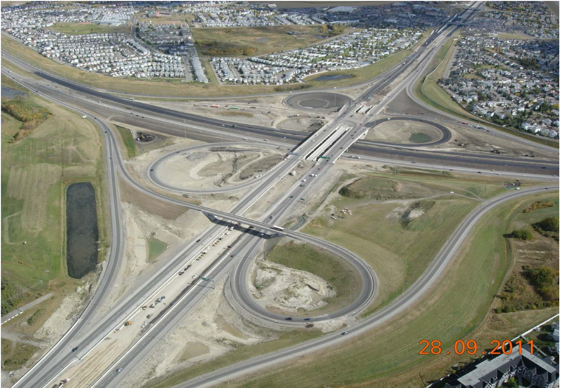
Stoney Trail / Crowchild Trail Interchange Looking Northeast September 2011
