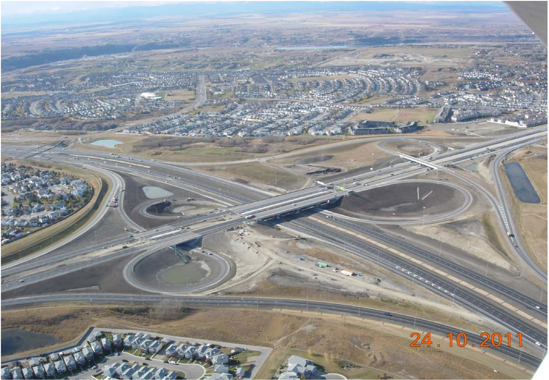
Stoney Trail / Crowchild Trail Interchange Looking Southwest October 2011
