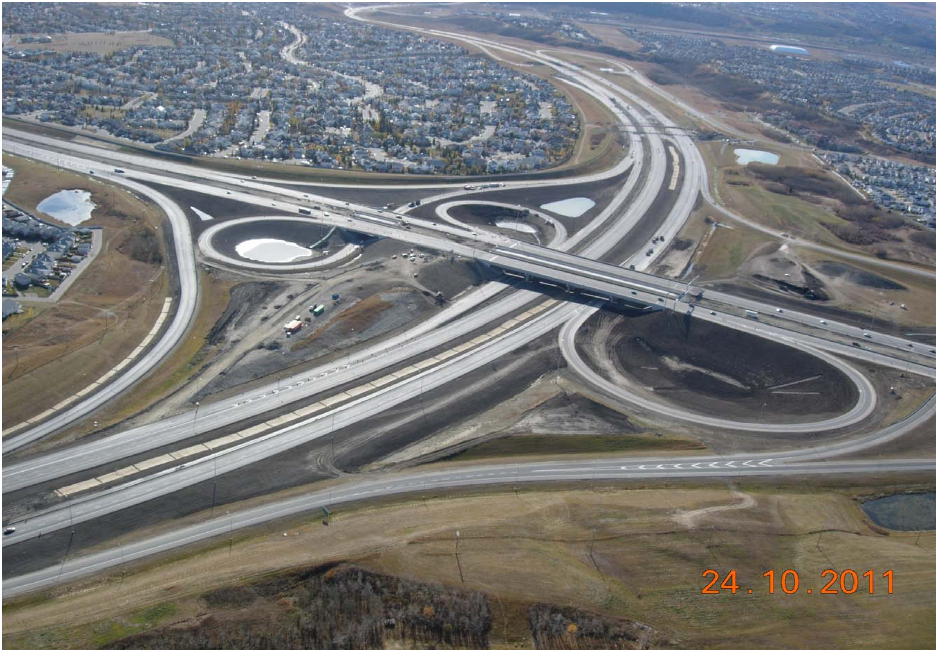
Stoney Trail / Crowchild Trail Interchange Looking Southeast October 2011
