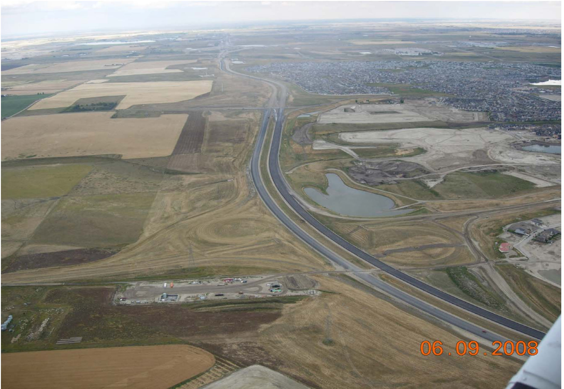
Stoney Trail / 14 Street to Harvest Hills Boulevard NW Looking East September 2008
