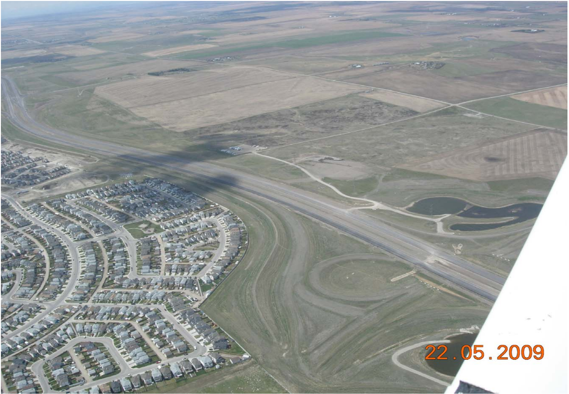
Stoney Trail / 11 Street NW to Harvest Hills Boulevard Looking Northwest May 2009
