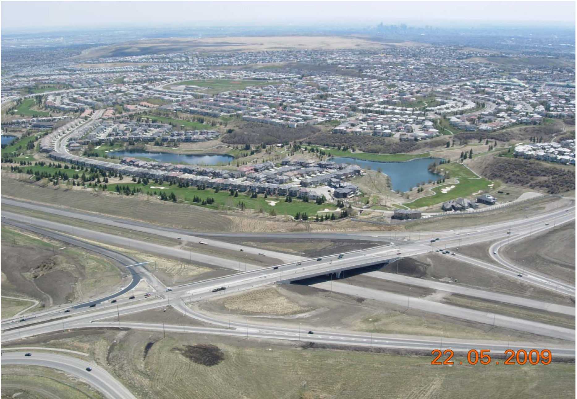
Stoney Trail / Sarcee Trail Interchange Looking Southeast May 2009
