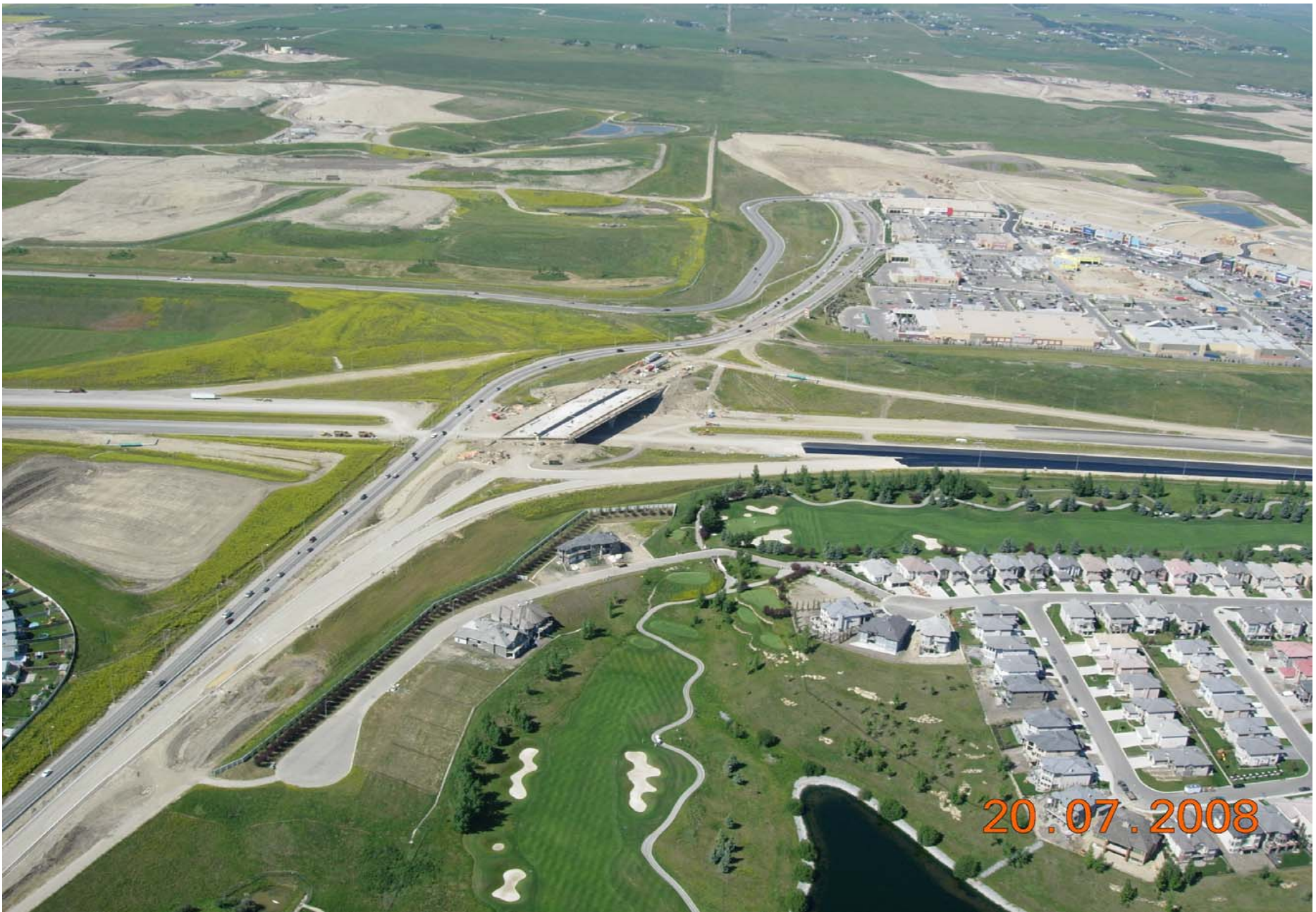
Stoney Trail/Sarcee Trail Interchange Looking North July 2008
