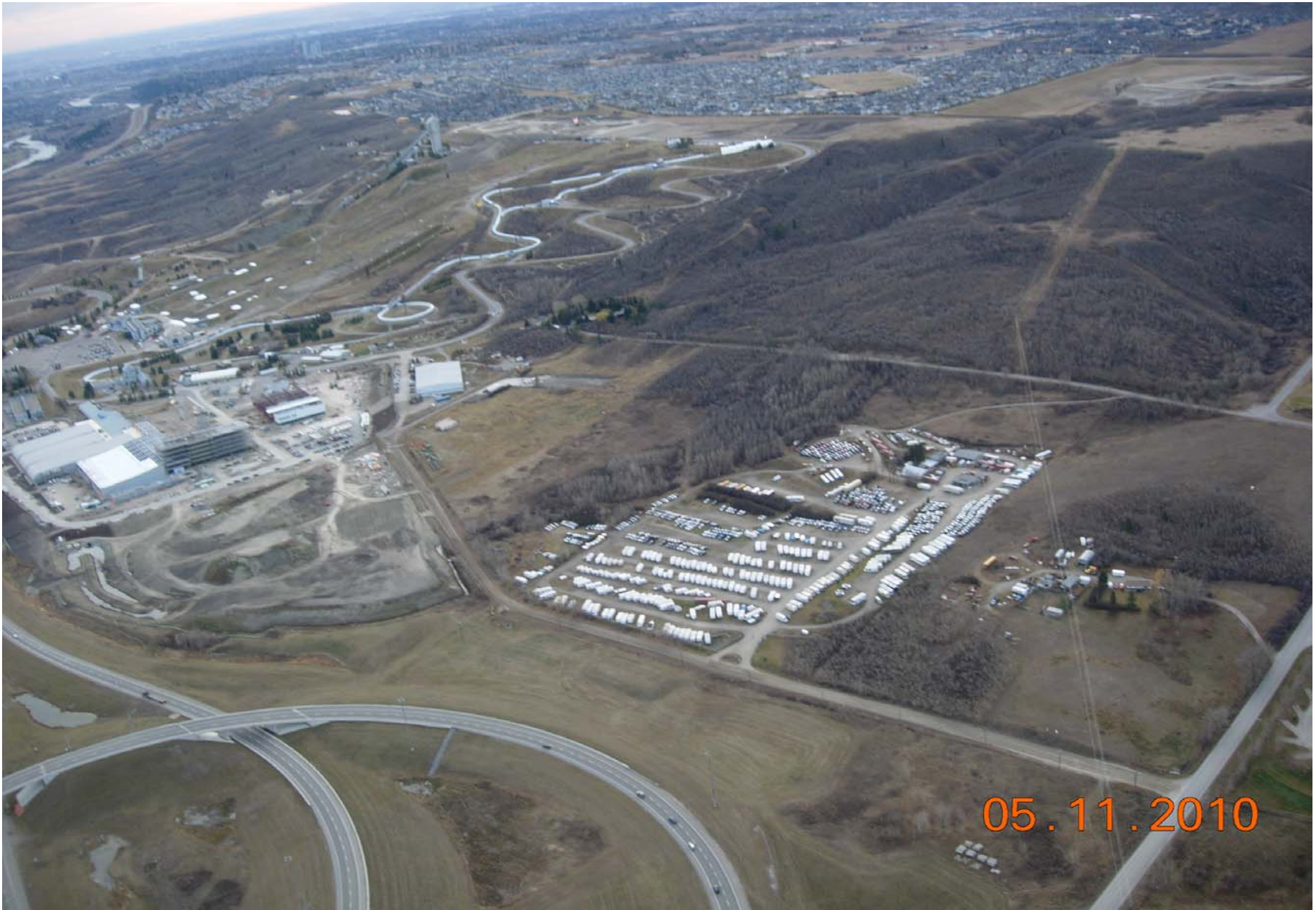
Stoney Trail / 16th Avenue NW Interchange Looking Southeast November 2010
