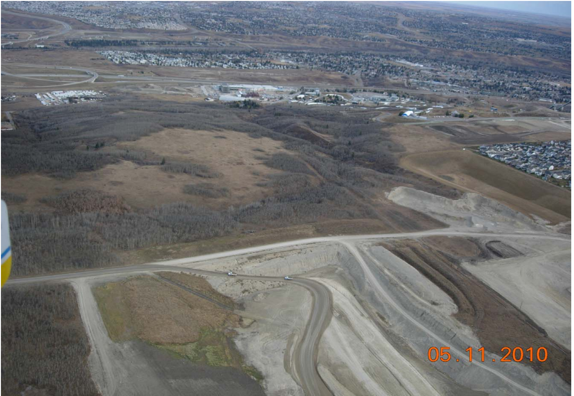
Stoney Trail / 16th Avenue NW Interchange Looking Northeast November 2010
