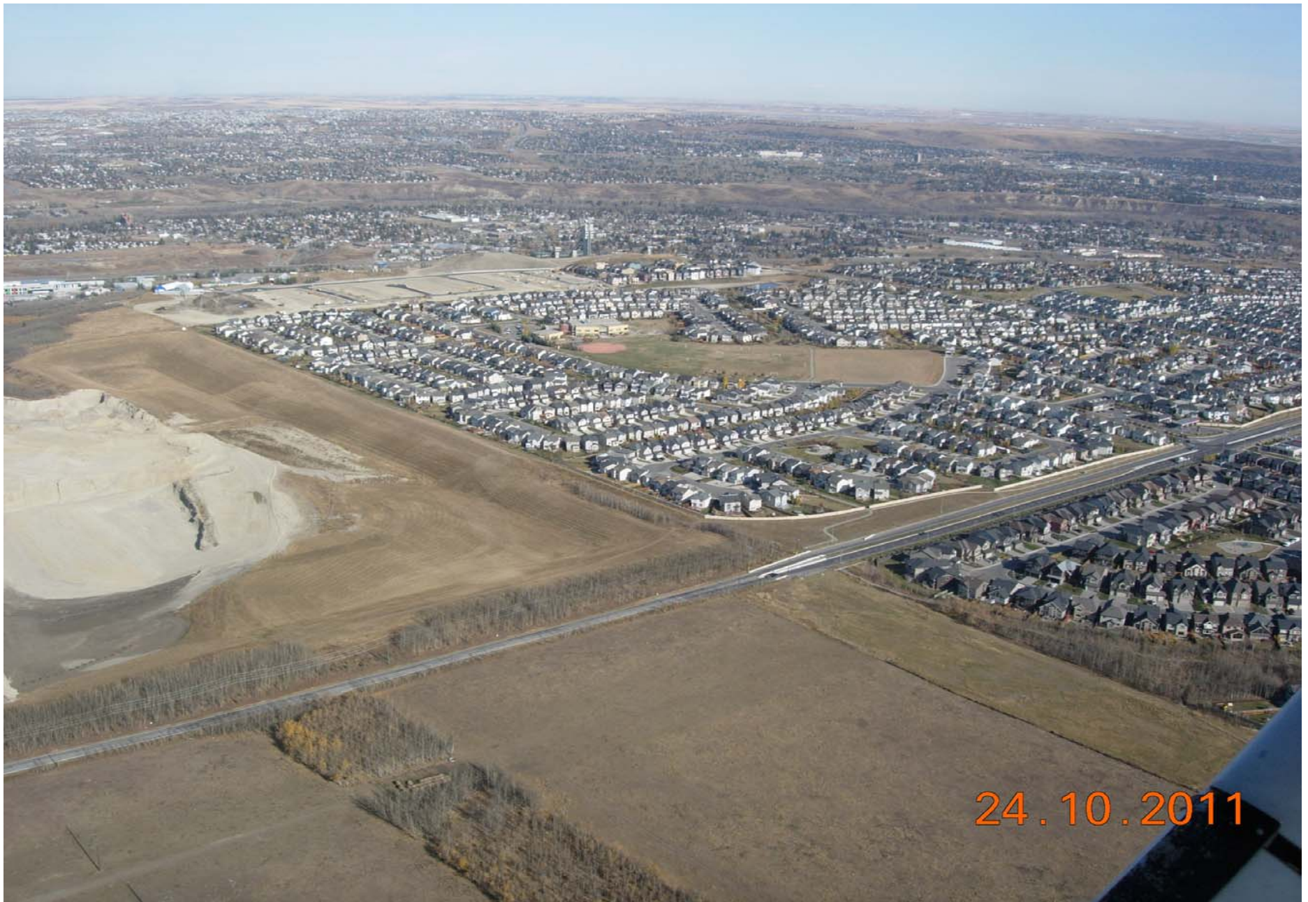
Stoney Trail / Old Banff Coach Road Interchange Looking Northeast October 2011
