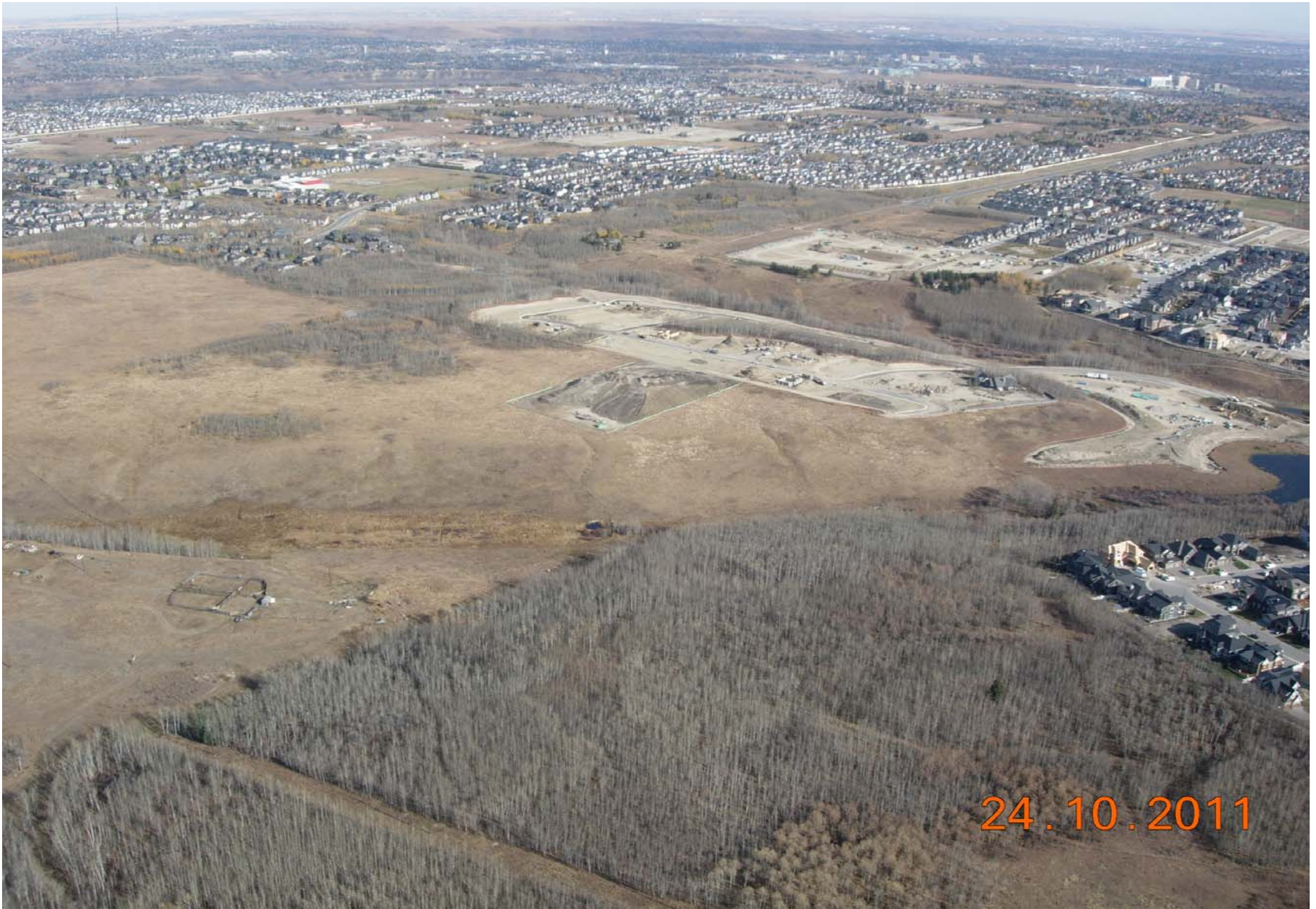
Stoney Trail / Bow Trail Interchange Looking Northeast October 2011
